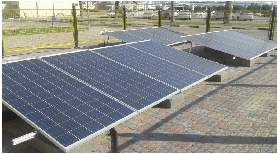
Figure 1. PV Modules Assembly at Nizwa College of Technology
